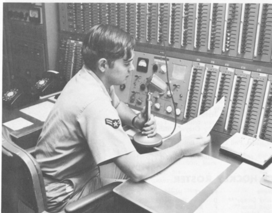
BUTTONS! BUTTONS! — Airman First Class Jerry Pugh reads an announcement over the public address (PA) system in Fairchild Hall, the Air Force Academy's academic building. The panel in front of Pugh contains 540 switches, one for each classroom, laboratory, auditorium and hallway in the six-story building. Pugh is one of two 1876th Communications Squadron technicians who operate the Fairchild Hall PA system and others in the cadet gymnasium, field house, Falcon Stadium and Cadet Chapel. No other communications squadron in the Air Force operates such an extensive PA network.
